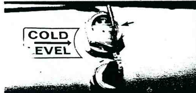
Figure 6-8. Surge Tank Sight Gauge.
